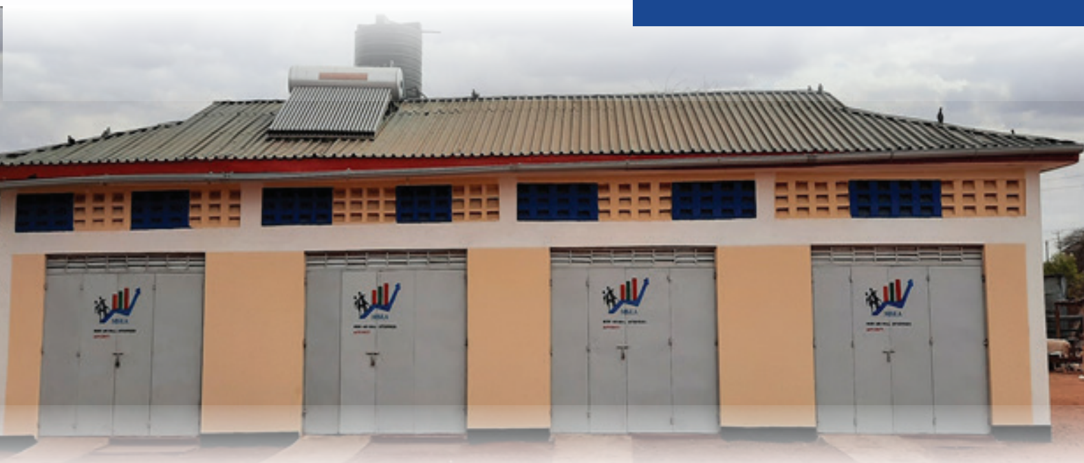
Enterprise Development Centre (EDC) - Wajir East
