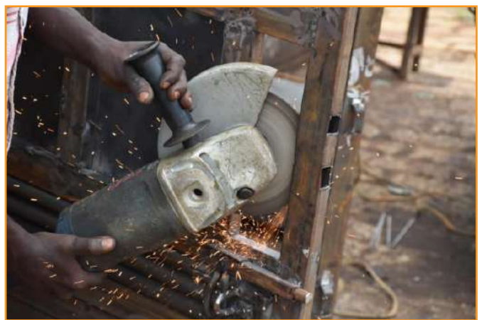
Welding in Meru town Juakali worksite.
