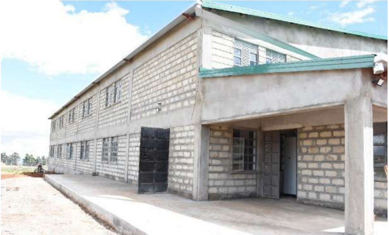
Current status of Timau Potato Cold Storage & processing facility.
